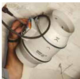
Carry out the wiring connections.
