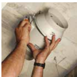
Place the impeller and motor assembly.
