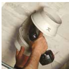
Fix the support bracket.
