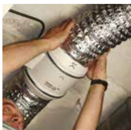
Connect the ducts.
